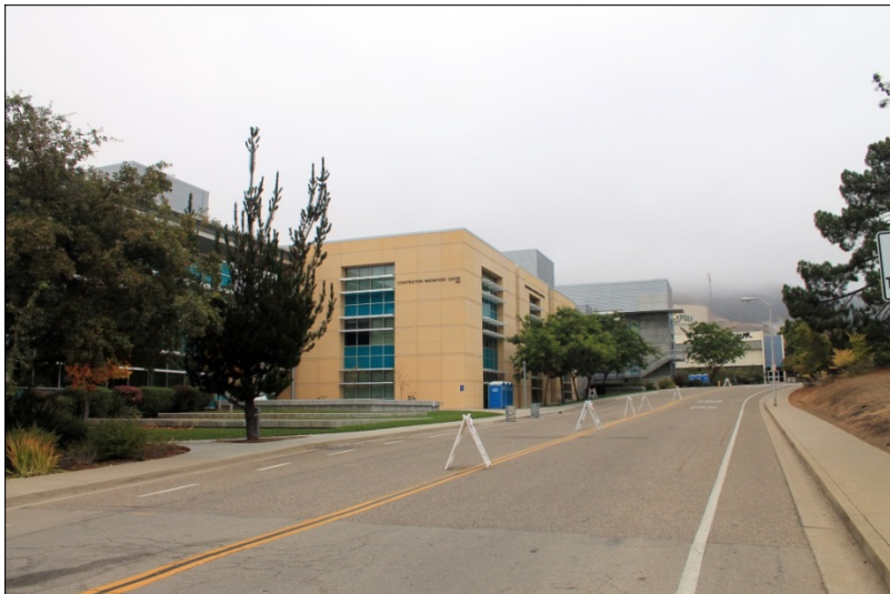
Photo 4.1-1. View of existing buildings near the campus core.
