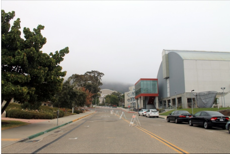
Photo 4.1-2. View of existing campus buildings along Perimeter Drive in the general vicinity of the project site.
